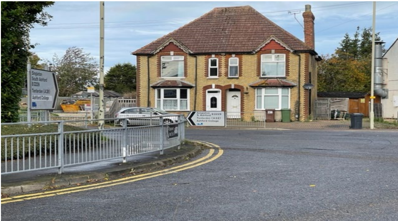
Figure 2: Photograph showing the pair of semi-detached dwellings
